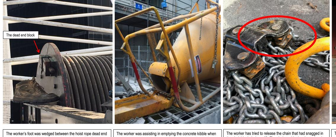
clamp on the side of the winch, and winch frame. The force caused a serious injury to the worker's right foot eventually resulting in a toe being amputated.
