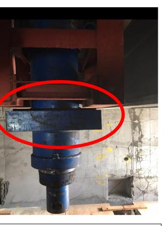
The worker was assisting the jumpform installer when he placed his fingers between and the truss and the jack. The sudden movement of the jack resulted in his ring finger being crushed. The tip of the finger was eventually amputated.
