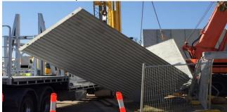
Tail-swing Clearance and Crane Setup Sufficient clearance to slew is obvious, yet often overlooked. The panel installation sequence and position of temporary panel bracing, (props) often causes issues here. Also, the Crane needs to be of adequate capacity with a current Cranesafe Green Sticker and set up on suitable ground with adequate timbers or mats.
