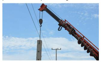
The dogman himself cannot be the spotter as his job is to control and land the load, which of course, involves looking at the load and hazards around it rather than up in the air at the boom. It's even more important on pick and carry cranes as they can come into contact with electrical hazards by not only luffing up but by traveling with the load (especially backwards).
