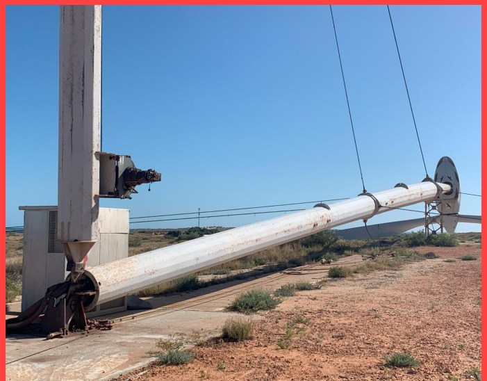
Vergent Wind Turbines installed at Coral Bay, Western Australia – offering a design that does not require a crane for maintenance (excluded from these statistics).
