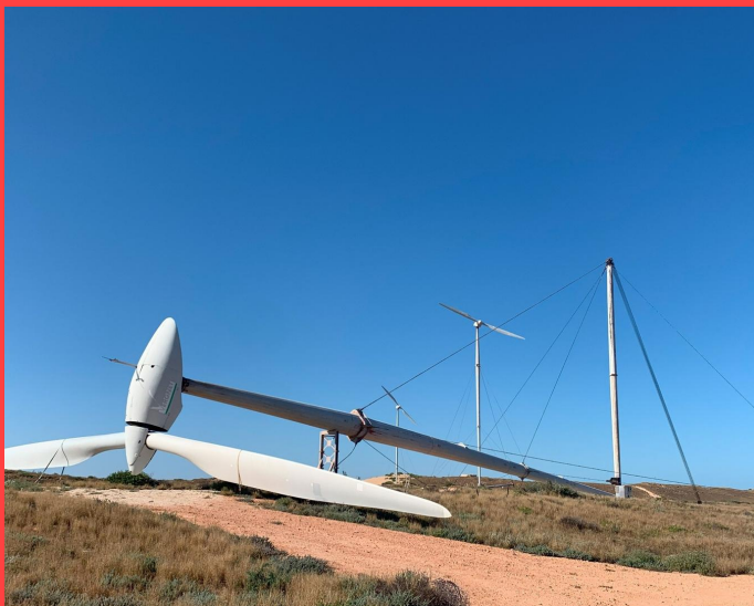
Vergent Wind Turbines installed at Coral Bay, Western Australia – offering a design that does not require a crane for maintenance (excluded from these statistics).
